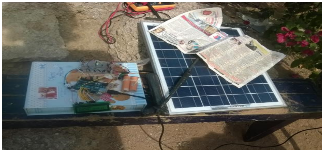
Figure 11: A dusted panel with reduced output voltage and activated wiper mechanism
